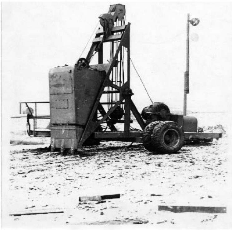
Fig. 1. Asymmetric vibration platform.
