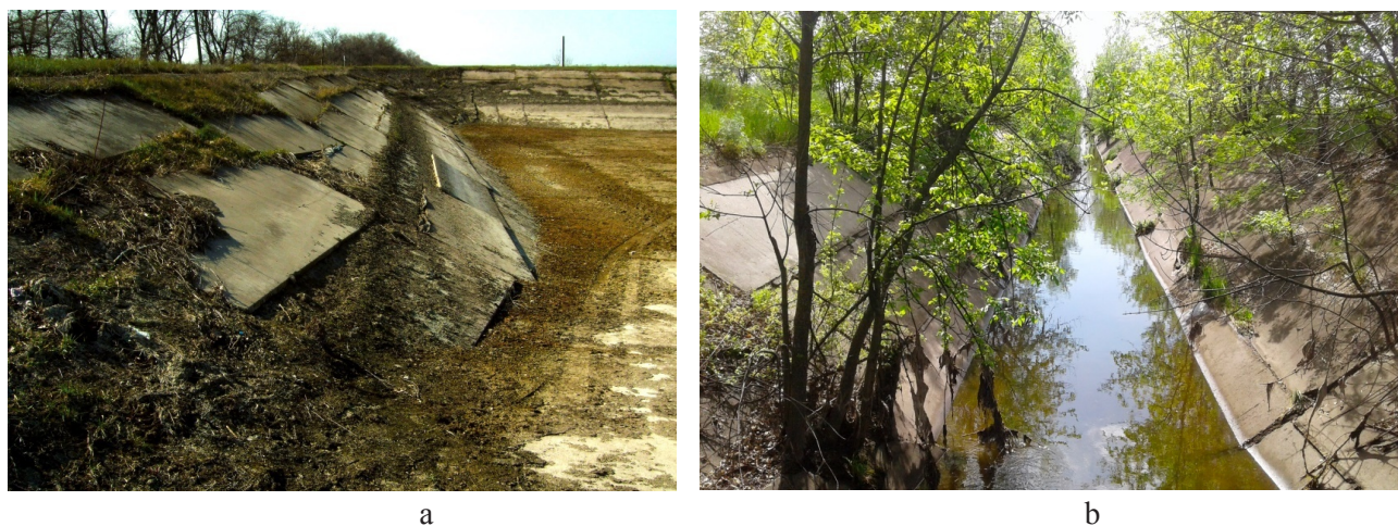
Fig. 6. Ruined areas of anti-seeping coverage at the current stage of technical exploitation of the structures: a – retention pond; b – main canal
