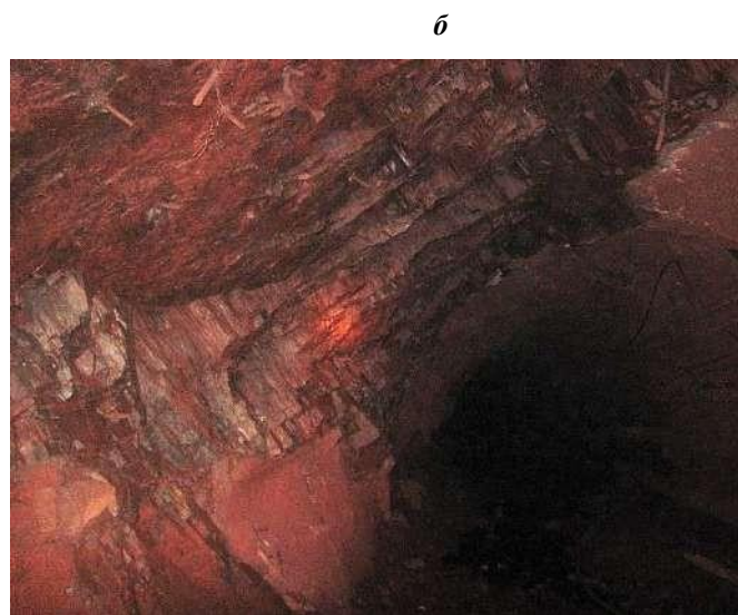
Fig. 1. Consequences of rock pressure manifestation in an unstable geological environment: (a) collapses of rocks of the hanging wall, when mining the ore from chambers; (b) chipping off and shear formation in the hanging wall drift of the 740 m horizon
